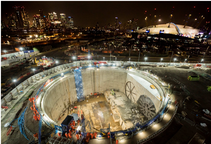
Fig.1 Rotation chamber Greenwich – TBM breakthrough overview
