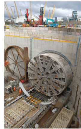
Fig. 3 TBM emerging from tunnel bore in Greenwich
