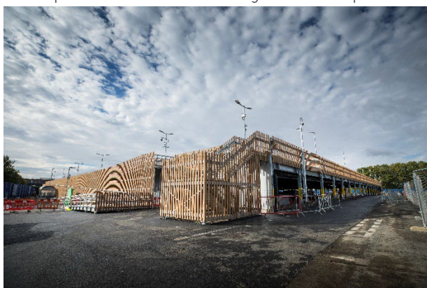
Fig.1 Decked car park
