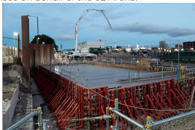
Fig.2 South Portal building roof slab – concrete pour
