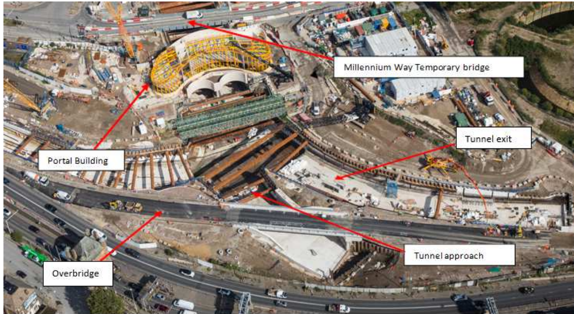
Fig. 1 The Silvertown Tunnel overview
