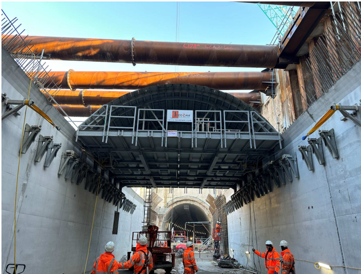
Fig. 2 Dome installation
