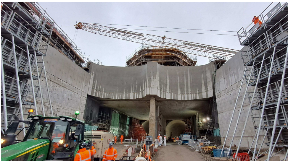
Fig.3 Open cut construction
