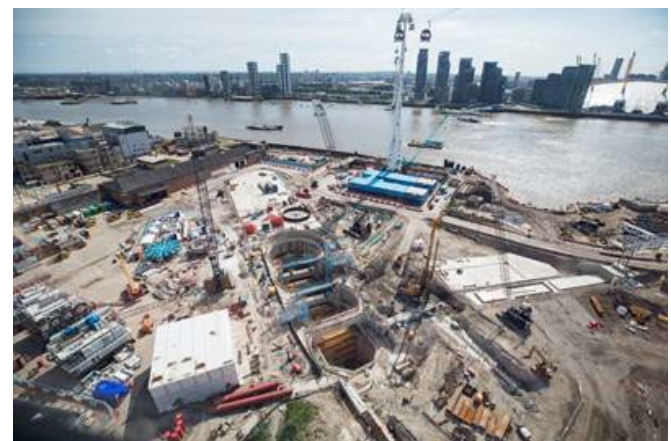
Fig. 4 Aerial view of the Silvertown Tunnel site, including the Launch Chamber
