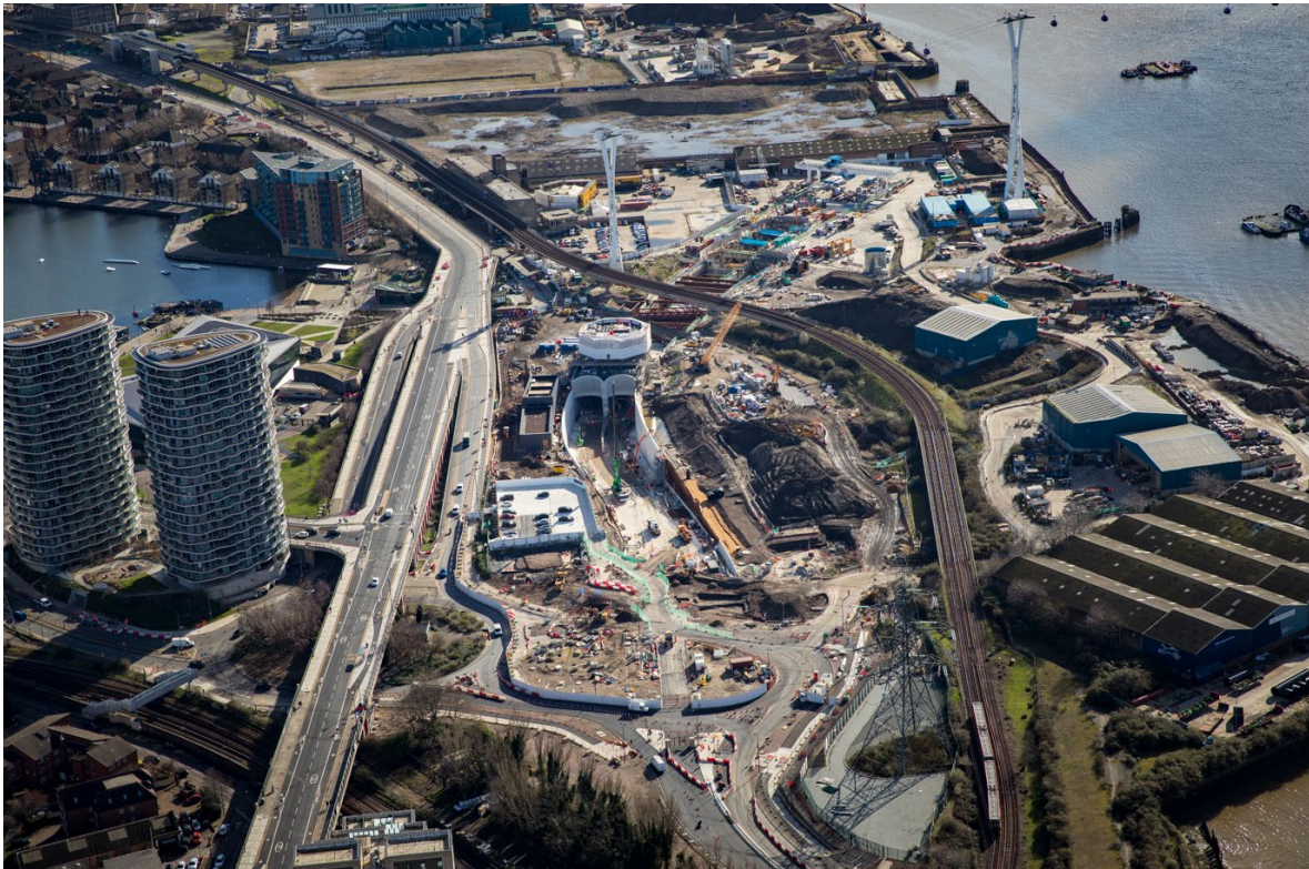
Fig.1 Greenwich site – Silvertown Tunnel
