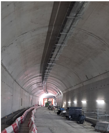
Fig.3 Inside the Cut and Cover Tunnel
