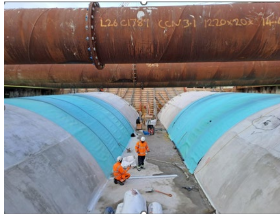
Fig.4 Waterproofing above the tunnel
