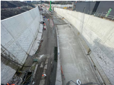
Fig. 5 'Open cut' structure looking north from the Portal building
