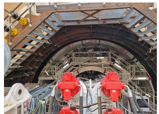
Fig. 3 First concrete ring installed
