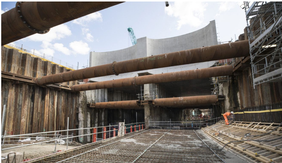
Fig.4 Open cut construction
